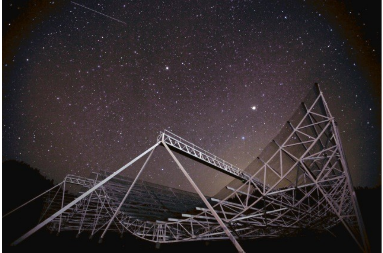
CHIME: Canada's radio telescope with no moving parts – all electronic!
