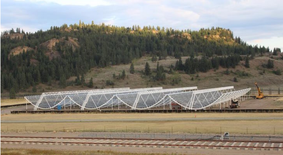
Figure 2.2: Full CHIME shortly after the construction of the fourth and final parabolic cylinder in fall 2015. Each dish is 20 m in the east-west direction and 100 m long. Unlike the Pathfinder, the cylinders are aligned with the celestial North Pole and should have true declination beams. There was also great care taken creating a smooth surface, since the Pathfinder’s relatively large surface RMS led to issues with its beams. Photo credit: Nolan Denman.
