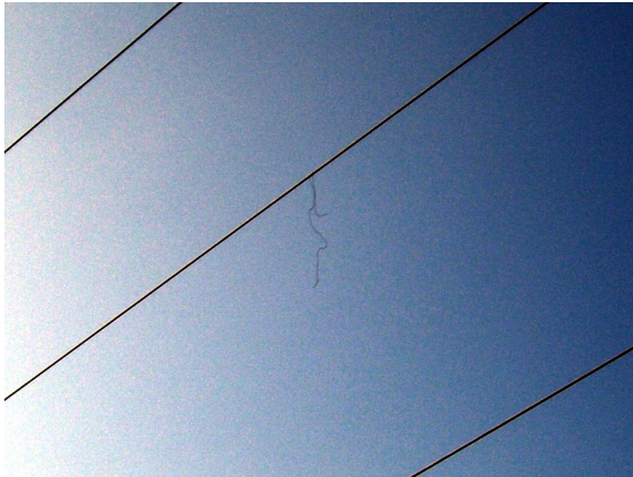
(a) Wire on 132 kV line
