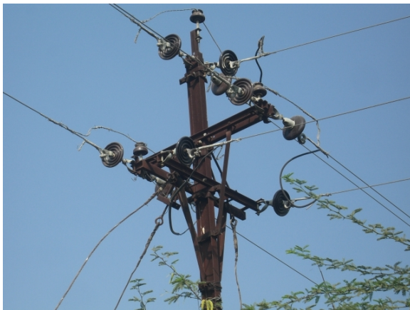
(c) Power line junction
