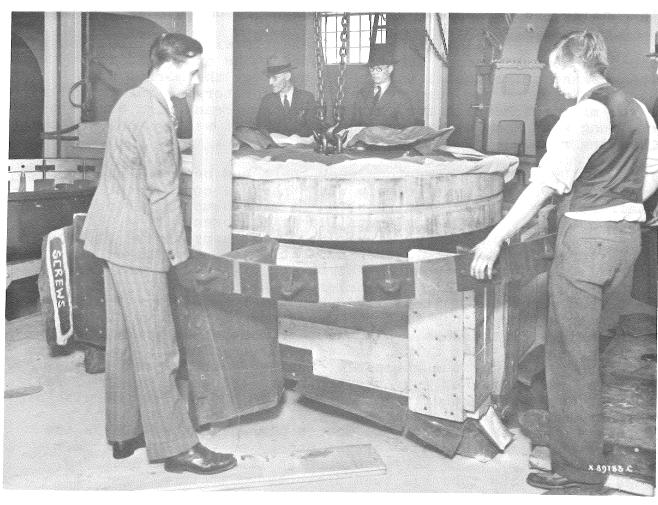
Lower: Frank Hogg and Jack Heard prepare to fit the supporting band onto the mirror before it is lifted into its cell at the left. Upper: Dr. Chant watches Dr. Young steer the eyes of the band towards the pins of the support system as the mirror is lowered into the cell. (Photos by Pringle & Booth, May 7, 1935)
