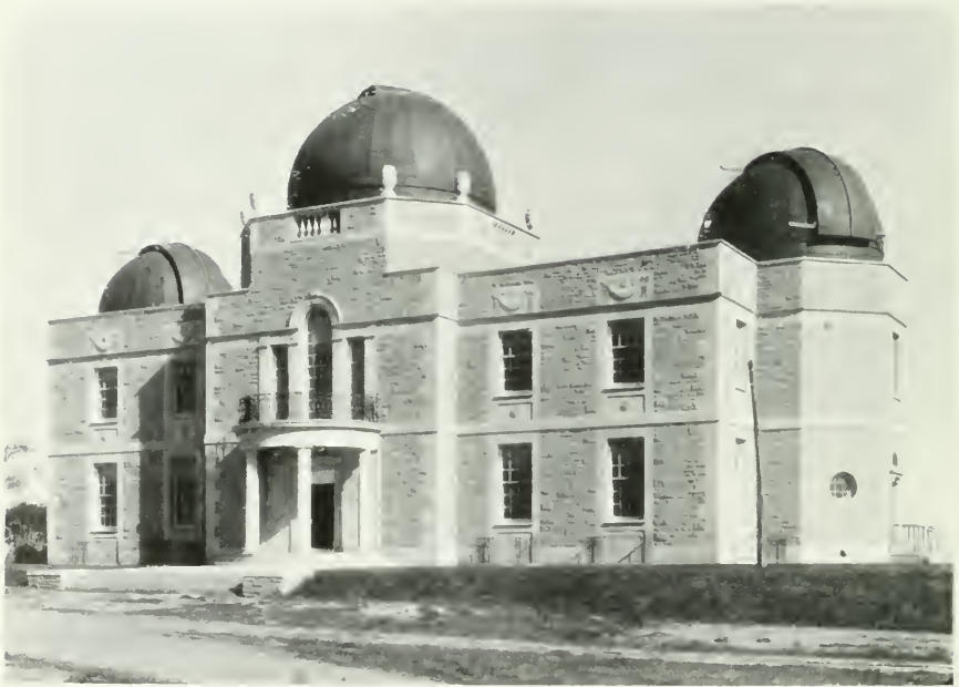
Front view of Administration Building from the west
