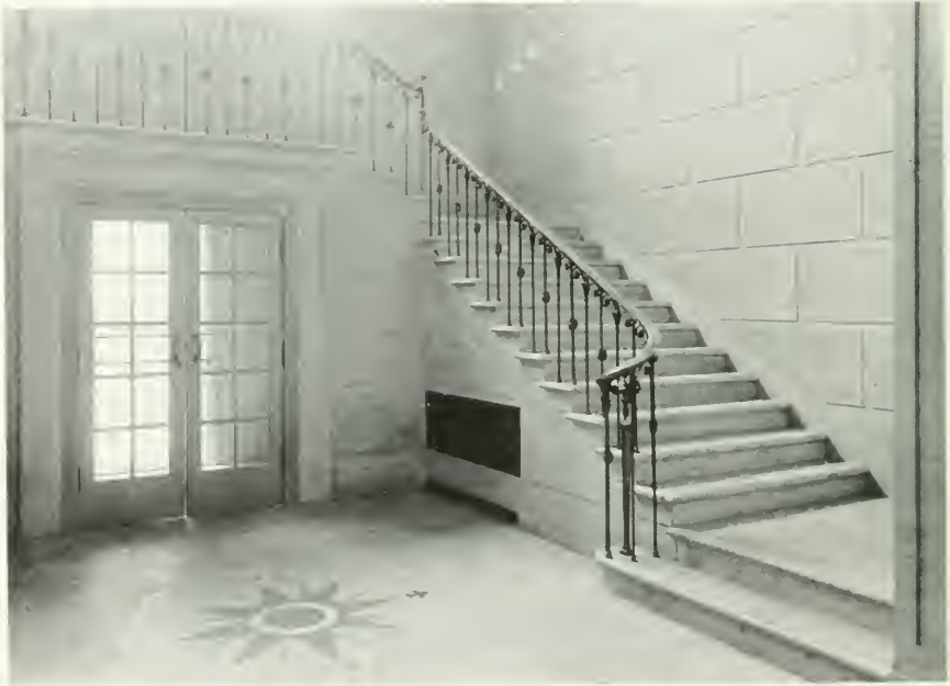
Main entrance Hall of the Administration Building
